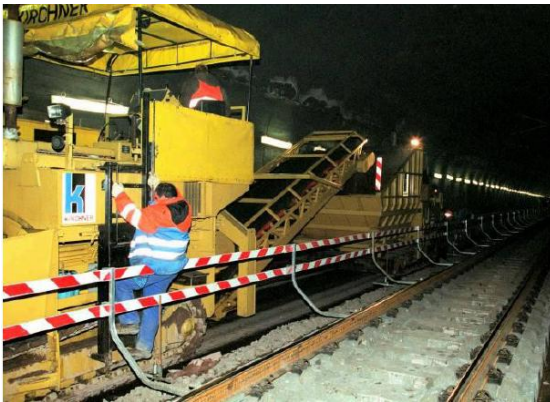
Figure 21. Paving with Asphalt
