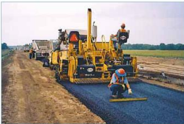
Figure 3. Placing Asphalt Underlayment on the BNSF Railway 'transcon' capacity improvement project
