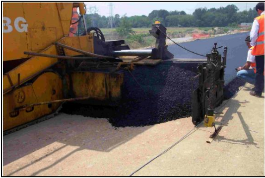
Figure 9. Placing of Asphalt Subballast (Teixeira, 2009)
