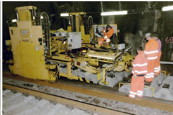
Figure 22. Installation of Concrete Ties
