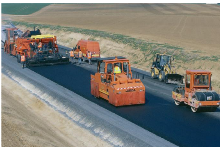
Figure 14. Asphalt Placement and Compaction (Faure, 2005)
